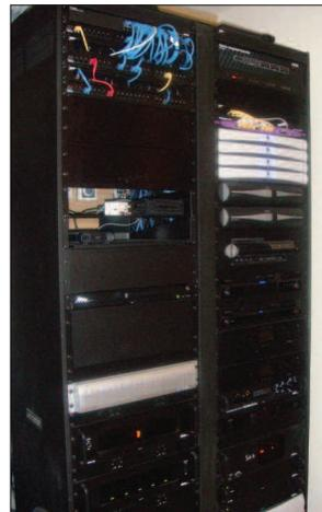
The Smart-e SNX-8x8+ was chosen for the project. Located in the hub of the house, the SNX-8x8+ delivers High Definition (HD) video to eight display screens around the property. All the sources are routed into the Smart-e SNX-8x8+ which are then scaled up to 1080p before they are switched through to the various rooms - so
